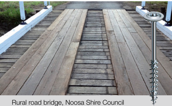
Rural road bridge, Noosa Shire Council
